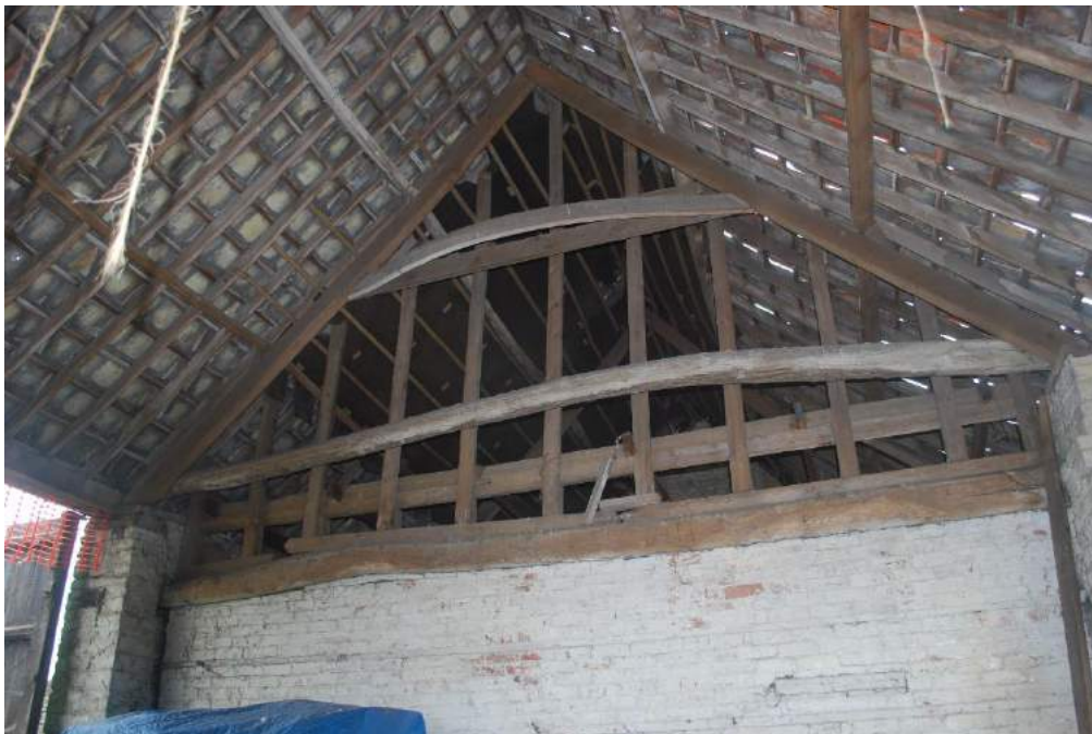
Figure 30: Bay 3, truss 3. The vertical timbers helped separate off the two end bays. The deflected collar, common to all trusses, is clearly visible.
