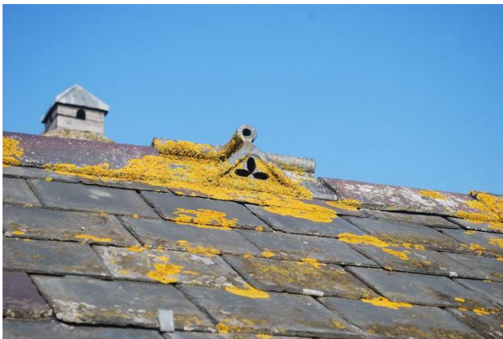
Figure 43: Four-ways roof vent (top of dovecote beyond).
