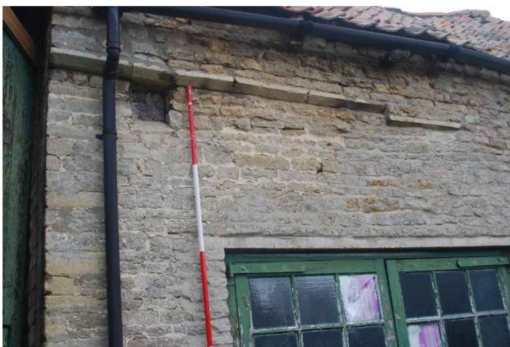
Figure 14: Re-used chamfered stone above garage door. Perhaps introduced when the upper courses were rebuilt at reroofing in the mid-19 th century.
