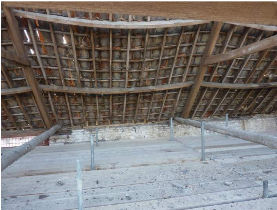
Addendum Figure 1. View east, centre of barn, showing flexed purlins.
