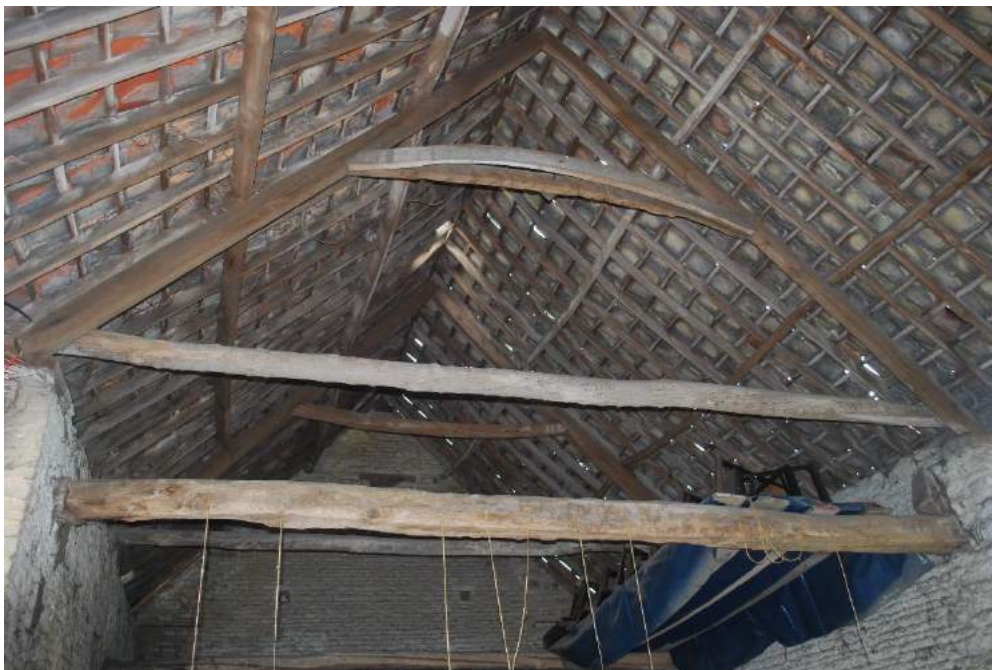
Figure 26: Looking north from bay 3, showing truss 3 (nearest camera) and truss 4. The generally lightweight nature of the roof timbers is clear. The larger beam set into the wall has no structural function. Such a beam is set beneath each of the four trusses.
