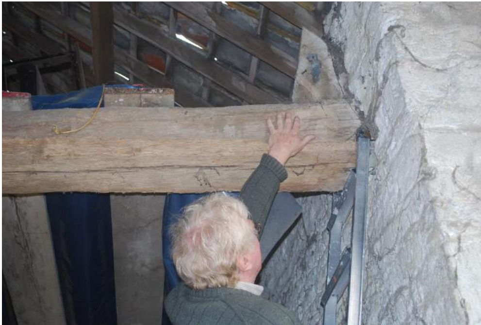
Figure 27: Large re-used beam beneath truss 3, east end, south face, to show sawn-off principal rafter.
