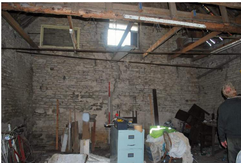
Figure 33: Bay 1, south gable wall. Note the large vertical crack to centre.
