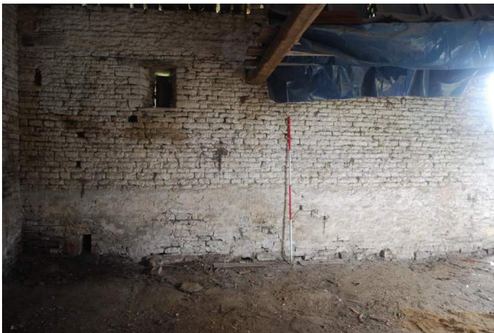
Figure 24. Barn, bays 4 and 5, east side, showing (a) splayed inner side of ventilation slit (b) plastered lower section of wall and (c) possible floor joists to right of ranging rod.
