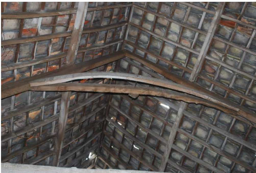
Figure 28: Truss 3, detail, showing deflection to collar (common to all four trusses) due to compression caused by the weight of the pantiles. An iron pin can be seen joining it to an inserted secondary collar.
