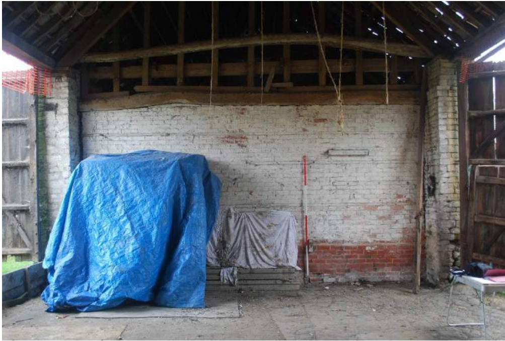
Figure 29: Bay 3, south wall. This wall is of mid-19 th -century date, and was inserted when bays 1 and 2 were separated off. Again, the beam above it which the brick wall abuts has no structural function.
