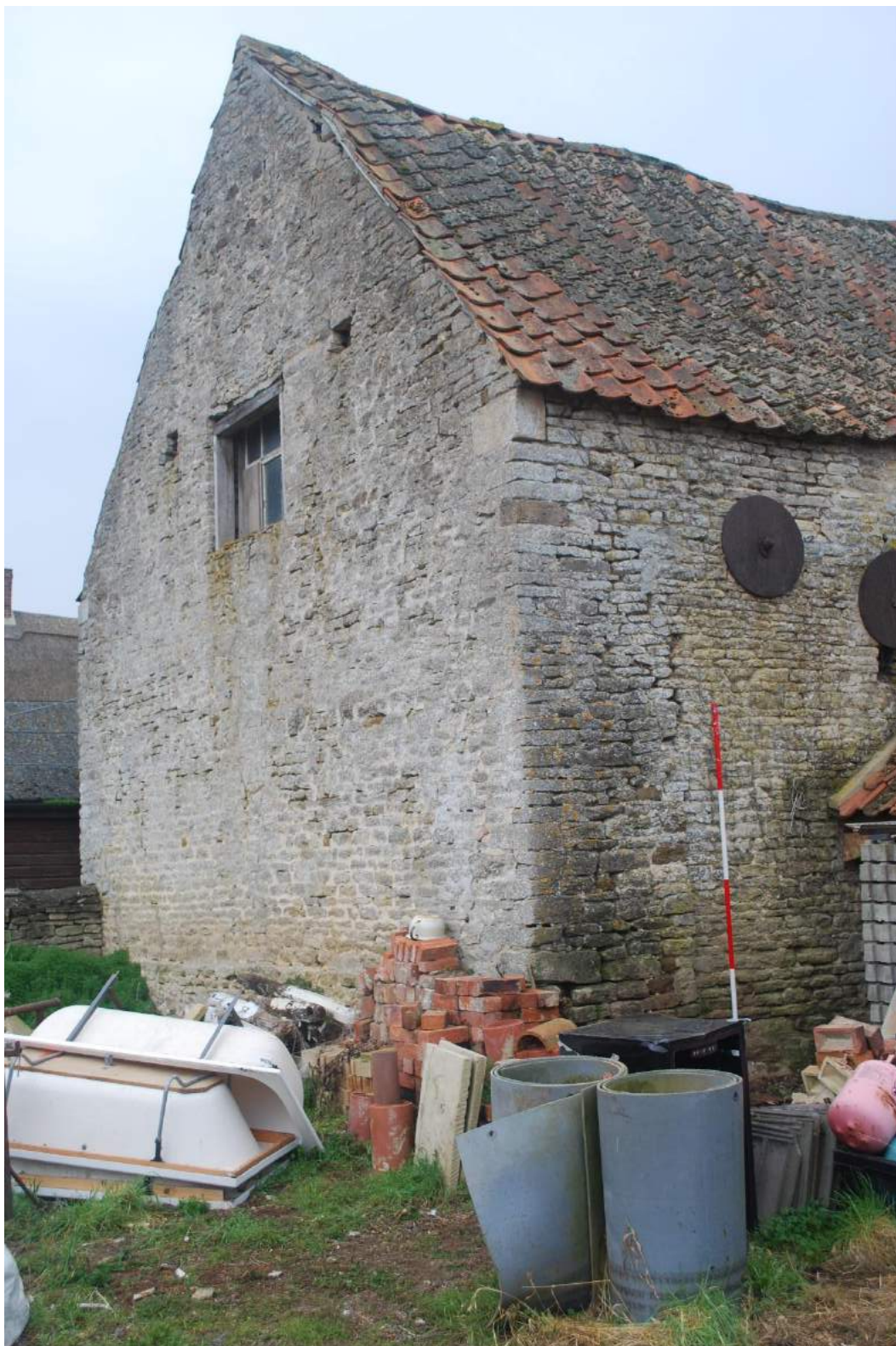
Figure 12: Barn, south-east corner. The gable wall, and the first metre of the side walls (see crack just to left of ranging rod), were rebuilt after a structural failure in the 19 th century. It is hard to assess if the two tie rods were inserted before or after this, or as part of the same repairs. Note ventilation slit under right-hand tie-plate.
