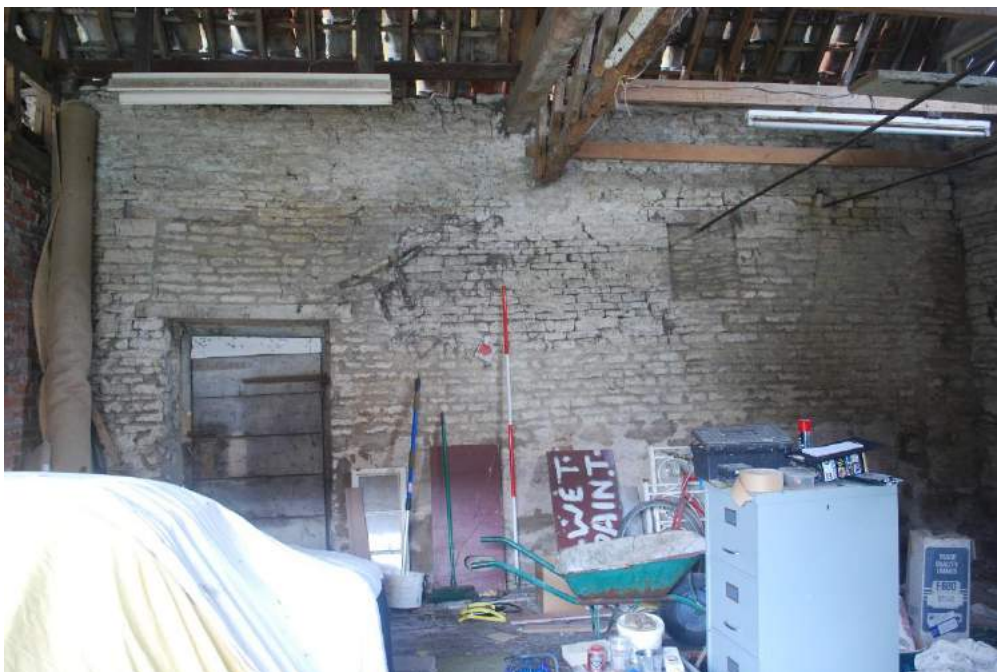
Figure 32: Bays 2 (to left) and 2, east wall, showing door with blocked window (perhaps a ventilation slit) above. Another blocked window (here certainly a ventilation slit) is to the right, now with a tie rod through it.
