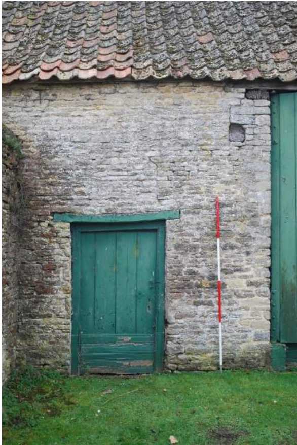
Figure 11: Barn, east side, bay 2. The door is a 19 th -century insertion. Its introduction led to the blocking of a window above, itself an insertion. Large-scale OS mapping shows bays 1 and 2 (which the door gives access to) were already divided off by the 1880s.
