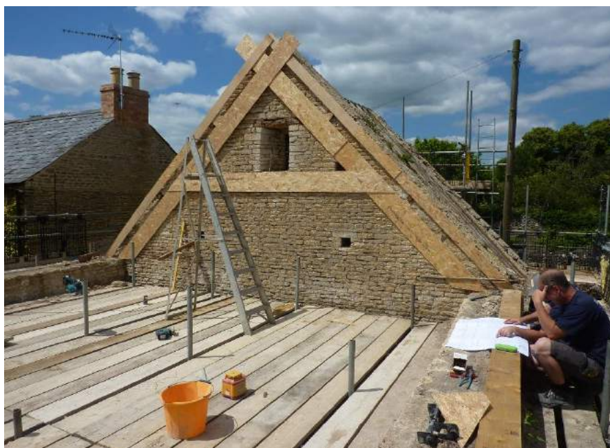
Addendum Figure 4. Rebuilding work in progress, July 2019, showing detail of upper part of south gable wall with splayed window and ventilation holes.
