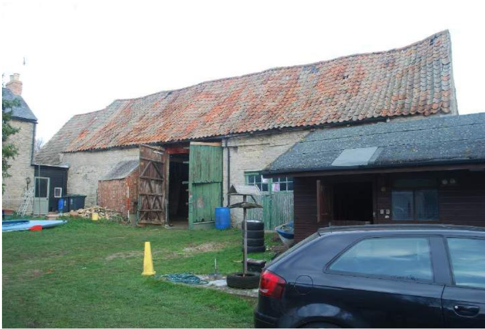
Figure 5: Barn, west side. Deflections in the roof due to the use of lightweight timbers can be seen.
