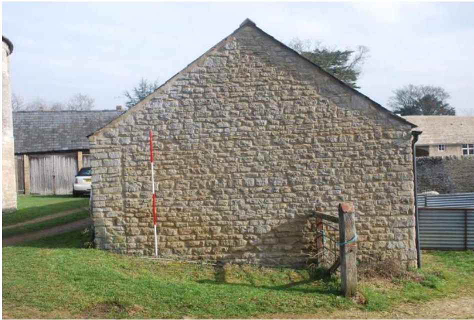
Figure 40: Stables, west gable wall. Note break in fabric to left of ranging rod.
