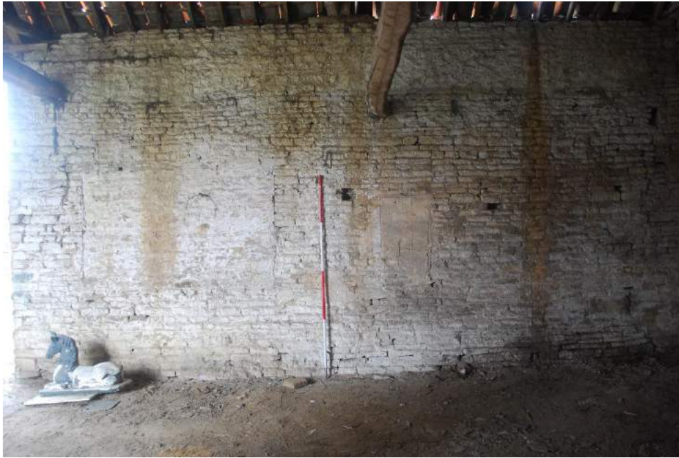
Figure 25: Barn, bays 4 and 5, west side, with blocked window left of ranging rod.
